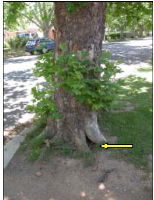
Plate 2: kerb and driveway showing decayed root
