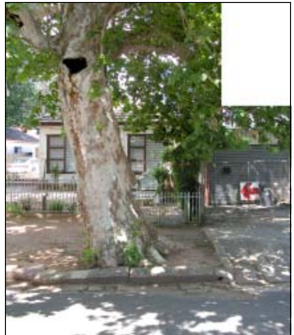
Plate 14: Damage to kerbing and driveway
