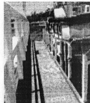
Jetty planking made from recycled plastic
